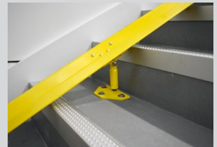
The wheeling ramps makes accessing the bike area much easier.
