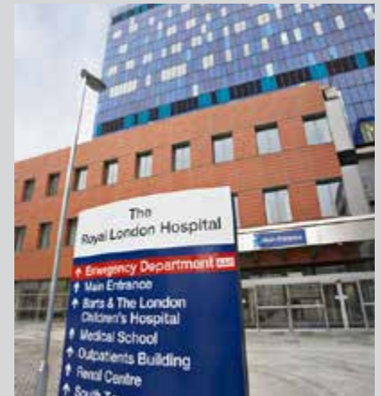
Cycle-Works were pleased to work with the NHS and Skanska on such a prestigious project.
