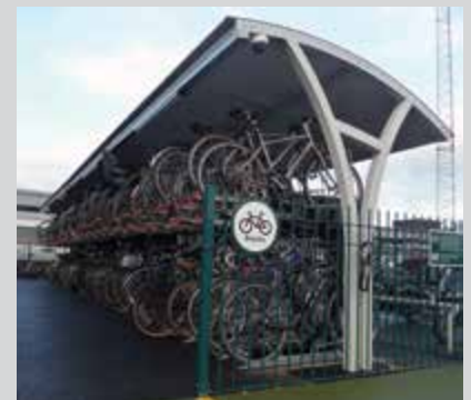
The Shelter is covered by 24 hour CCTV and features internal lighting.
