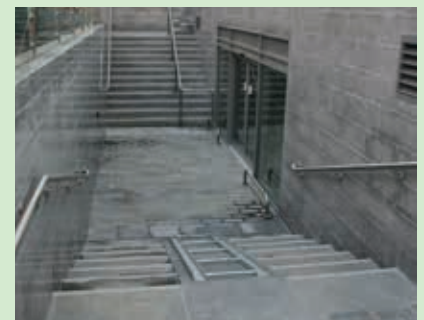
Wheeling ramps have been integrated into the design of the entrance.
