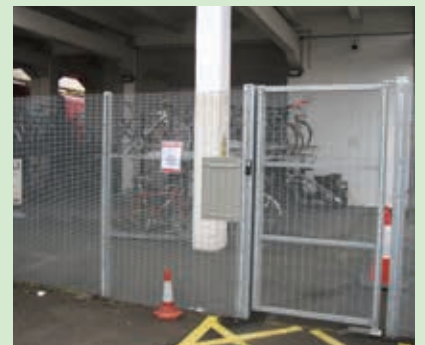
Cycle parking at Surbiton is now enclosed in an electronically locked compound.
