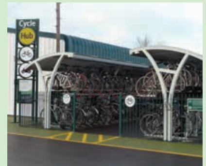
144 Josta 2-Tier Racks under the Cycle-Works Kennet Shelter
