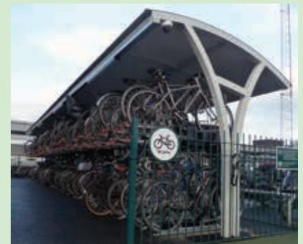
The Shelter is covered by 24 hour CCTV and features internal lighting
